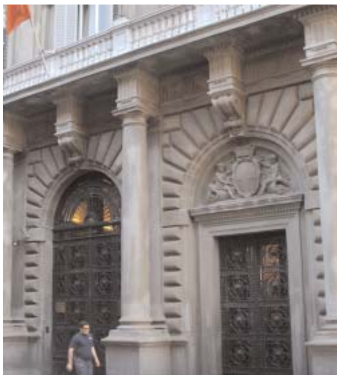
Headquarters of the Bank of Italy.
